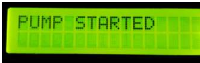
Figure 7.Displays status of pump Wind speed is not related with conditions this is only for indication purpose.
